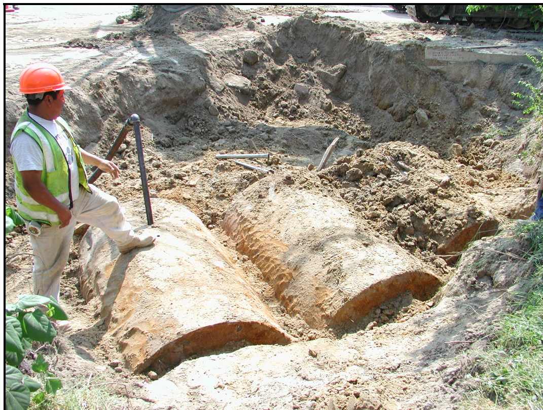
Figure 70. Underground Storage Tanks (USTs), Feature 13, uncovered in the northeast corner of the Town Park. View looking east (May 2007).
