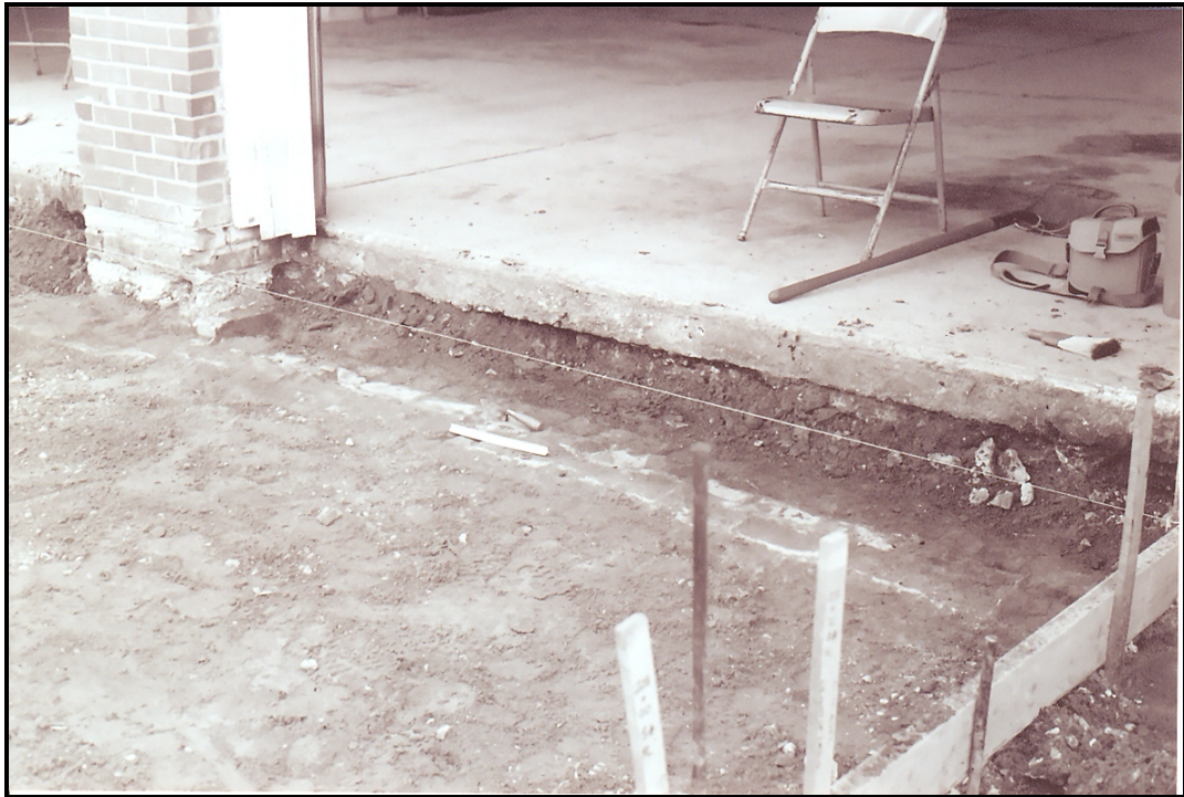
Figure 64. Brick foundation, Feature 7, exposed below the concrete sidewalk, south bay of the East New Market Fire Company, North Main Street. View looking northeast (August 2007).
